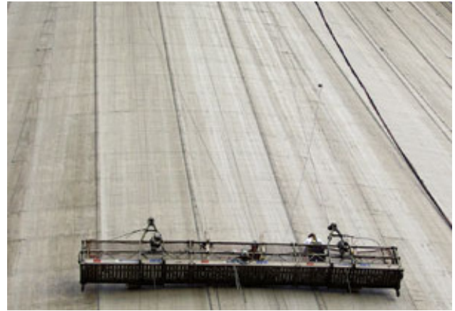
A utility had to cut cladding on a cooling tower and worried how far it safely could go. Analysis showed it danced in the wind but was safe.
